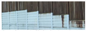
Photograph 1 - Unpainted hardwood causing tannin stains on concrete
